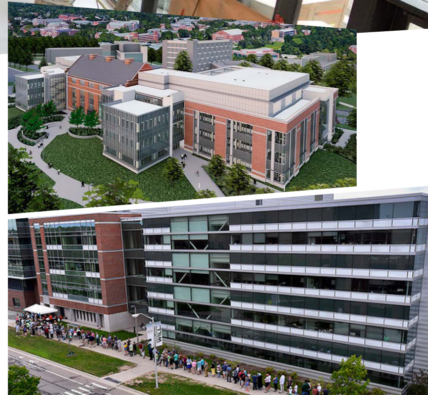
Top: Music students continue learning while construction takes place outside their classroom. Above: An artist rendering of the future STEM Teaching and Learning Facility. Below: Community members line up for tours of MSU nuclear physics facilities.
